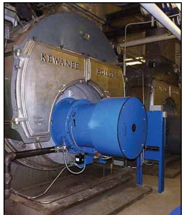
A FD68 burner retrofit gives serviceable boilers a new lease on life with better efficiency and reliability.
